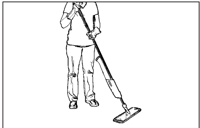
Figure 5. Applying floor finish with Flat Mop (optional).
